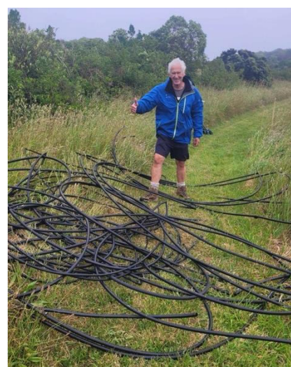
Steve with the removed irrigation piping! Image by Will.
