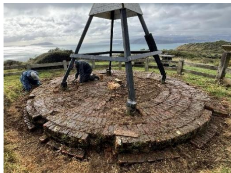
Work nearly complete. Photo Colin Munn
