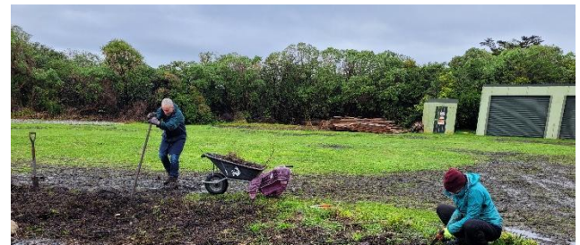
The demolition site Photo Bronwyn
