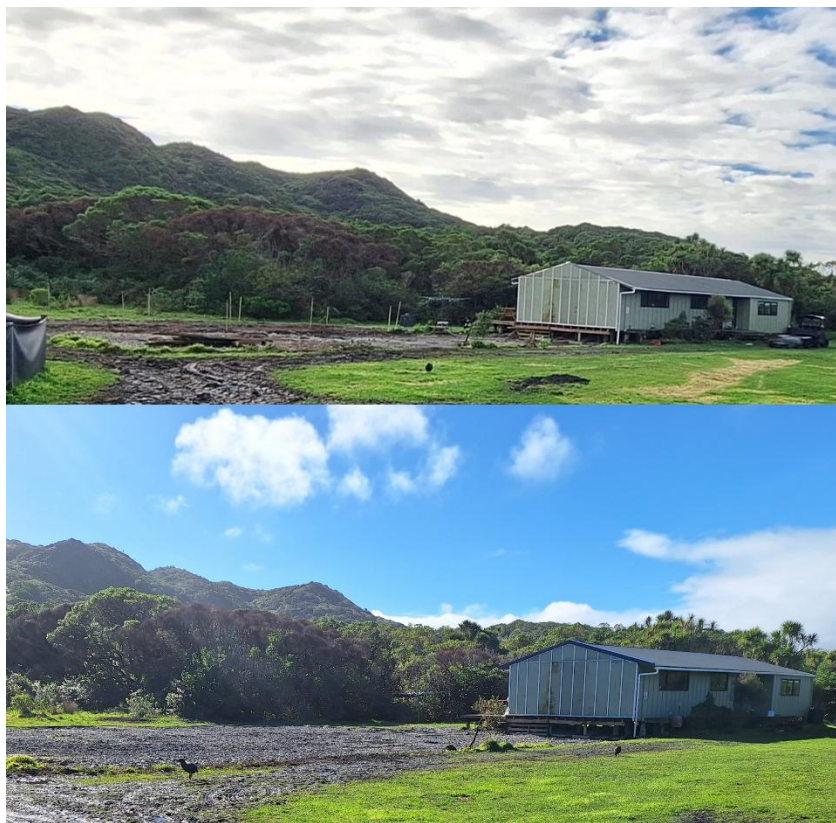
Huge changes to the demolition site Photo Colin Miskelly
